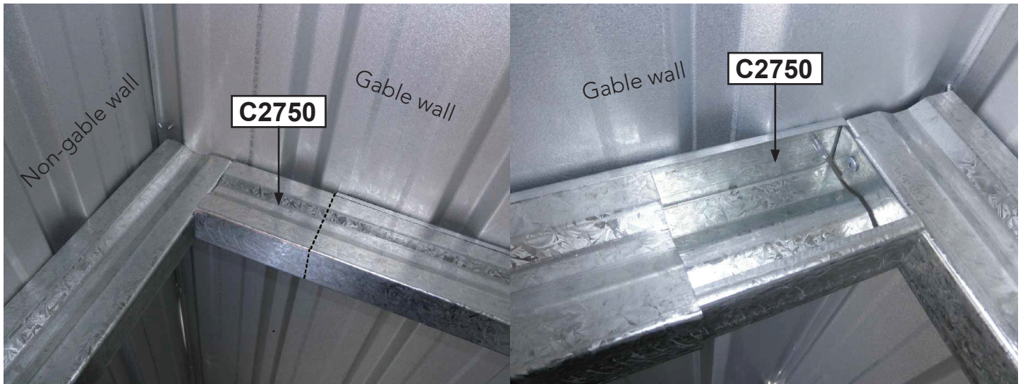
Previously installed wall bracing on the left and new gable wall bracing on the right.
