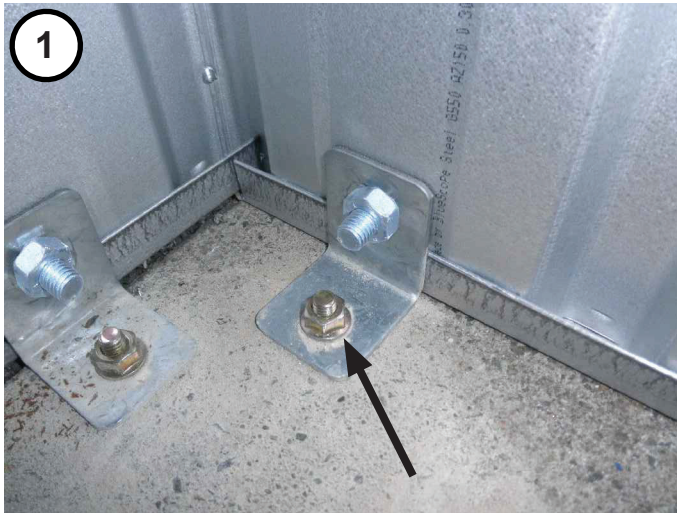
Inside view of typical anchor.
